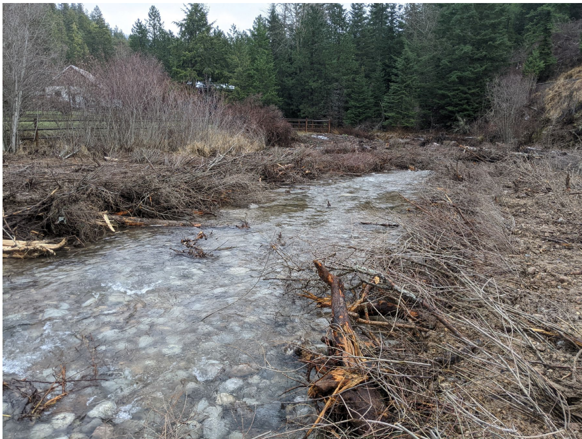
Photo 22: Post Construction. Installed Vegetated Wood Matrixes and constructed streambed downstream of property owner's structures. Facing downstream ( PXL_20201125_173543929.jpg )
