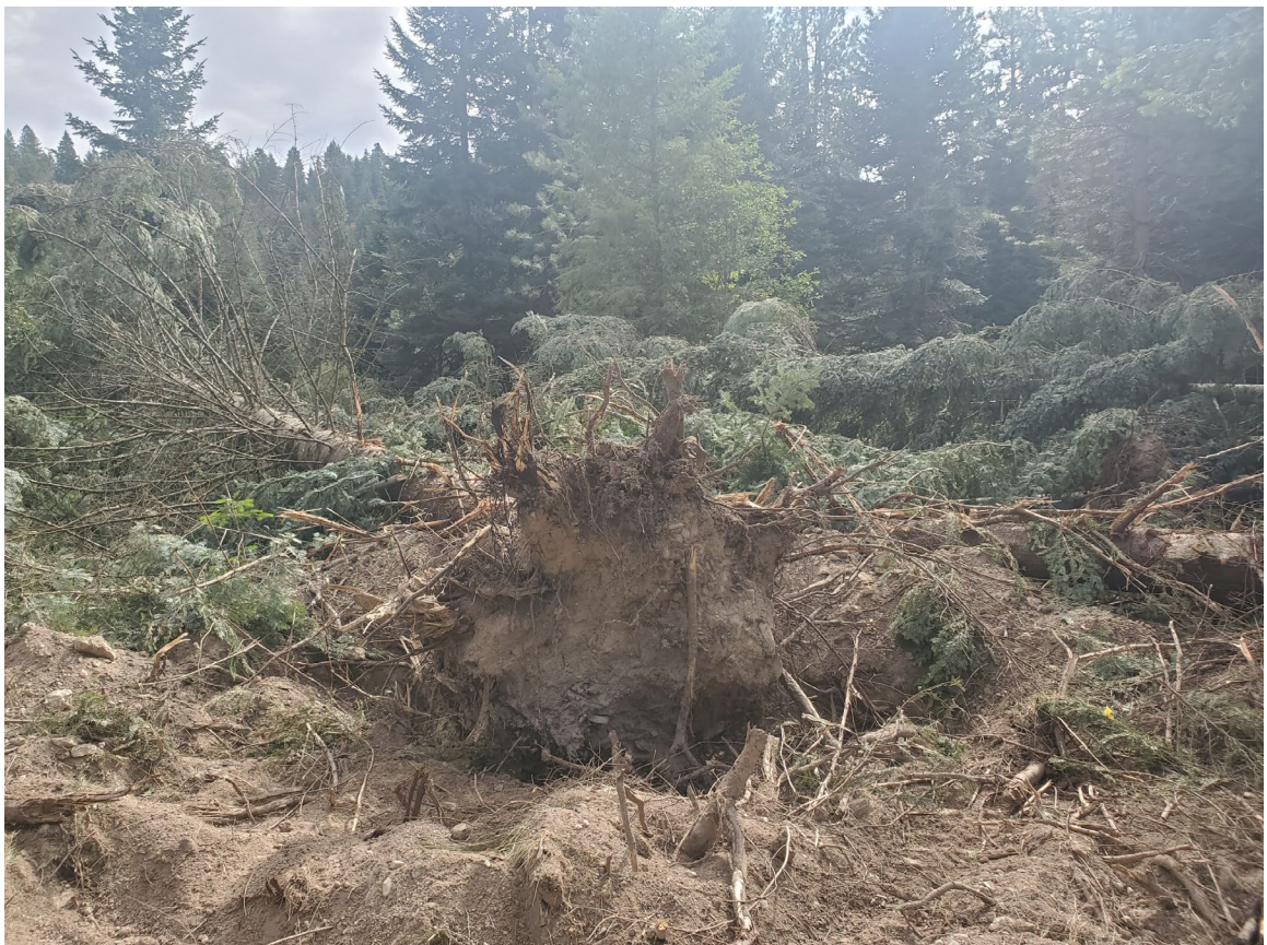
Photo 10: Construction. Collecting Category 1 wood. ( Cat 1 wood (a).jpg )
