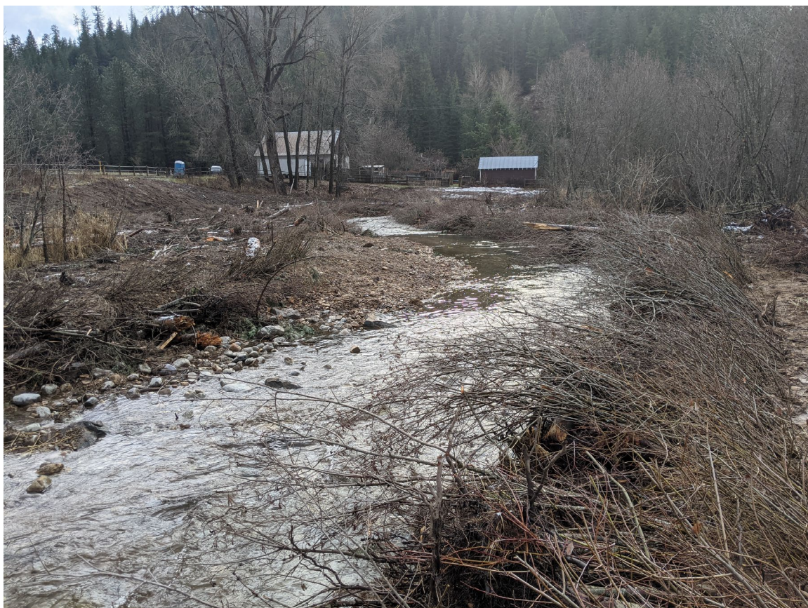
Photo 21: Post Construction. Installed Vegetated Wood Matrixes and constructed streambed upstream of property owner's structures. Facing downstream. ( PXL_20201125_172445806.jpg )
