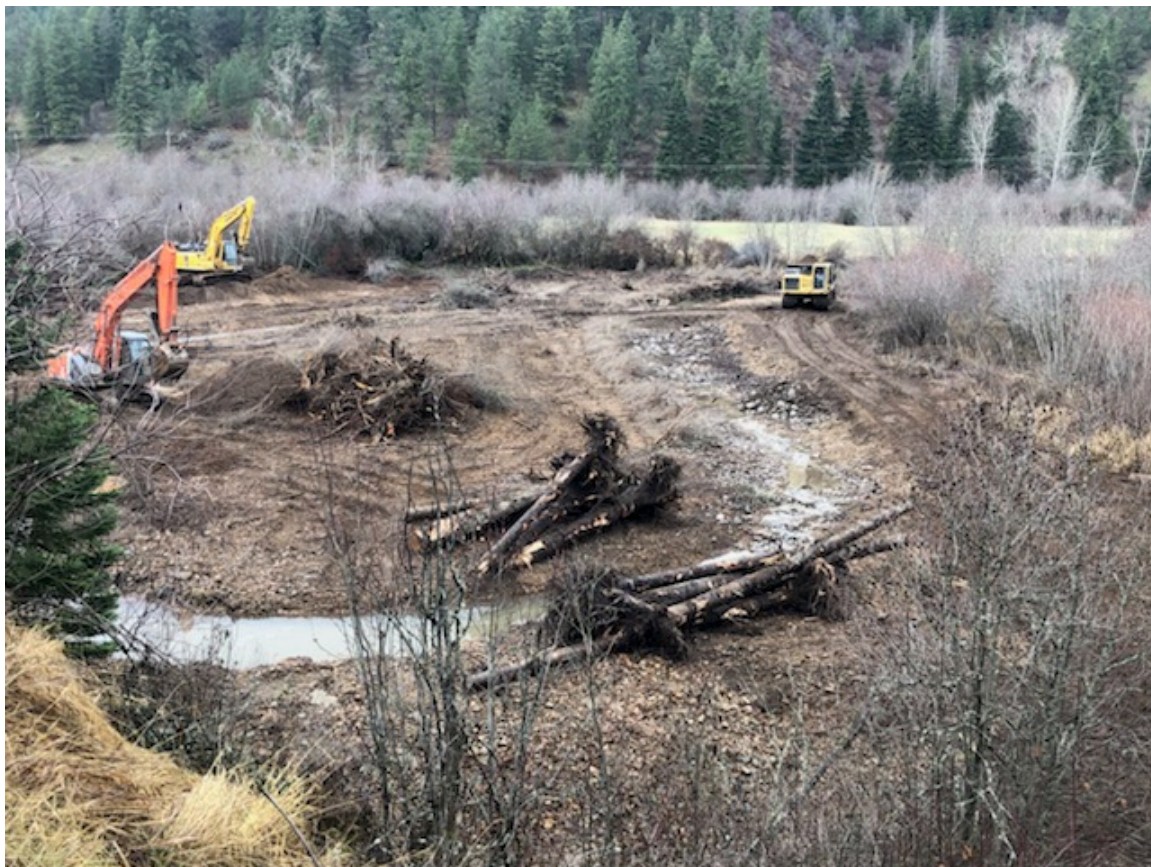
Photo 17: Construction. Recontouring of stream channel and floodplain enhancement, down stream of landowner property. Viewed from S Wolf Lodge Creek Rd. ( Road view.jpg )
