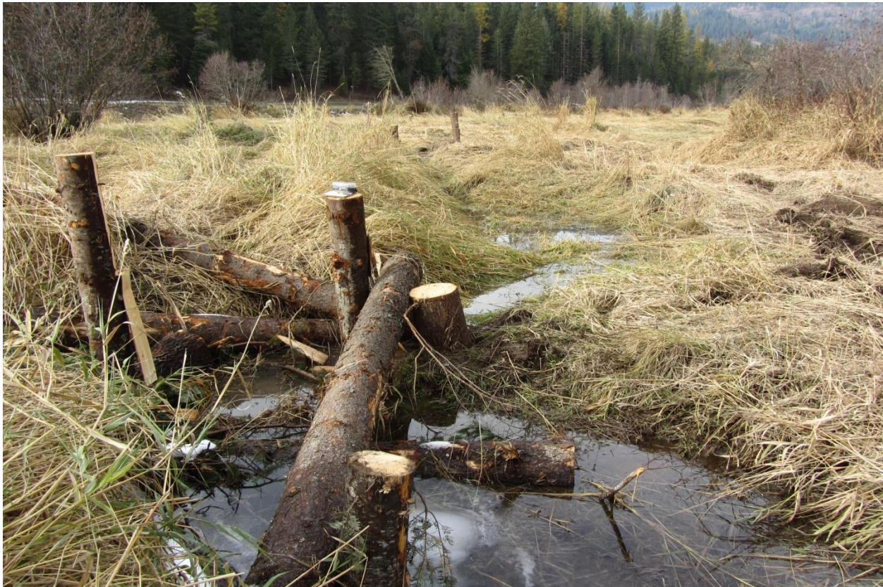
Photo 1. Instream wood placement in upper Lake Creek, October 2020.
