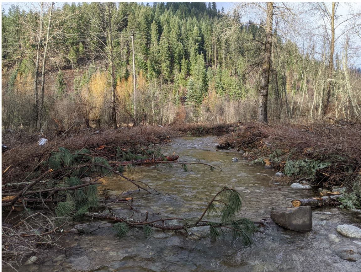
Photo 19: Post Construction. Installed Vegetated Wood Matrixes and constructed streambed upstream of property owner's structures. Facing upstream. ( PXL_20201125_172143597.jpg )
