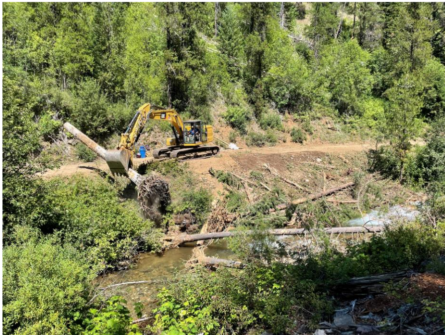
Post Dam removal at Red Ives
