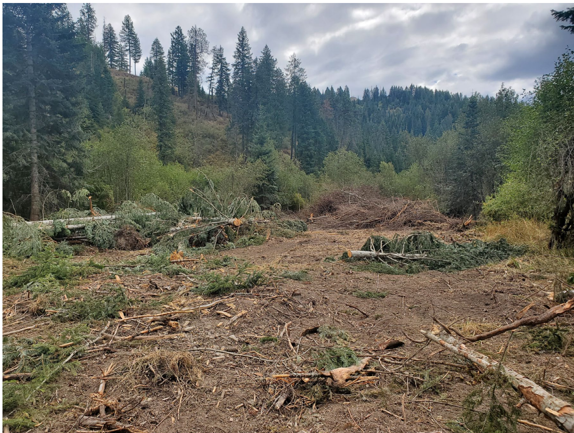
Photo 11: Construction. Staging area. ( Staging Area 1.jpg )
