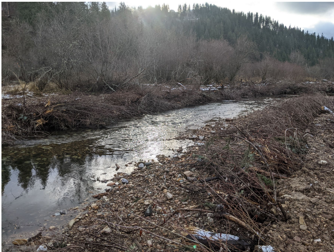
Photo 18: Post Construction. Installed Vegetated Wood Matrixes near upstream edge of project area, looking downstream. ( PXL_20201125_171322887.jpg )
