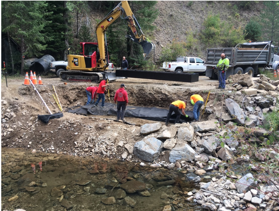
Install Bridge Footings
