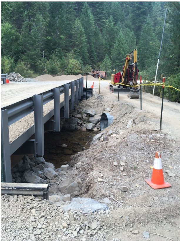
New Travel Surface Placed. Temporary Crossing Ready for Removal.
